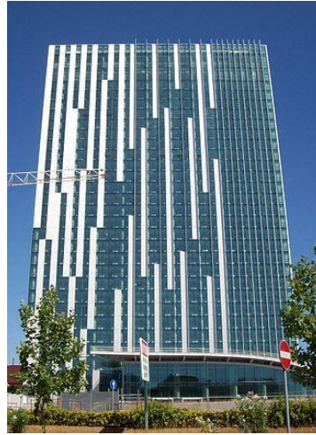
Figure 6. “Europarco” Tower in the EUR district of Rome (Photo by E.M. Mazzola)
